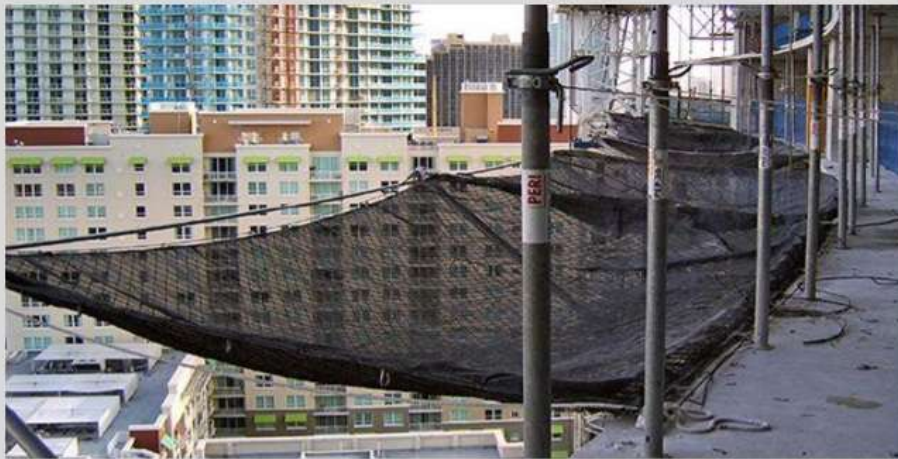
Construction Safety Net
